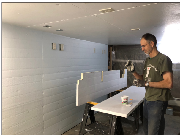
Don cutting insulation board for the fish room in 2021. Note the electrical outlets high on the wall and ceiling.
